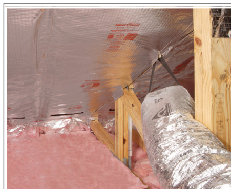
Radiant barrier installed onto under side of roof.
